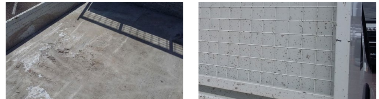
Trace of concrete or chemical product covering more than 1/4 of the surface of the load bed
