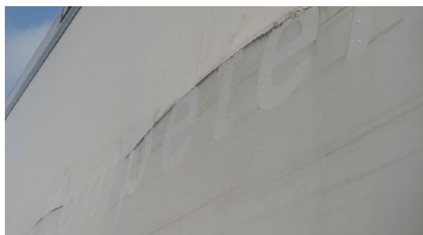
↻ Fibre side panels: Deformation on lower part, length of greater than 1 m NB: Replacement of the front panel of the underbody requires removal of the underbody.
